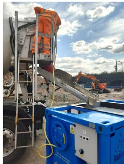
The solids will be caught in the Nappy Sack, the pH of the water will be reduced as it passes through the sack and drains into the sump where it returns to the tank, forming a closed loop.
